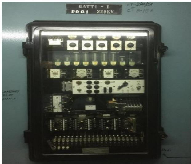
*Fig. 10. Distance Relay at 220 kV Grid Station Faisalabad.*
