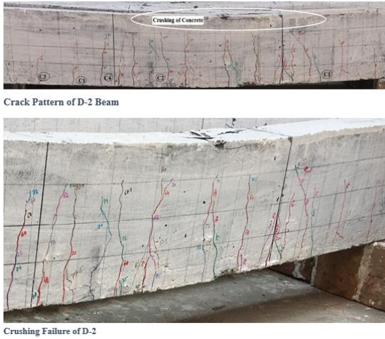
Fig. 10. Failure Pattern of Beam - D2
